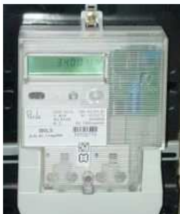
Solid state electricity meter.
